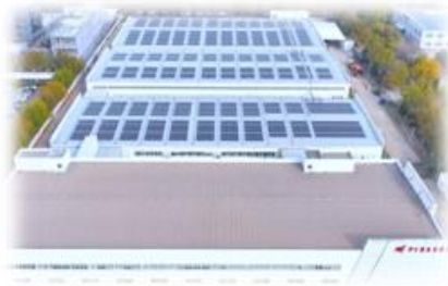
Solar power generation at Tianjin production facility
